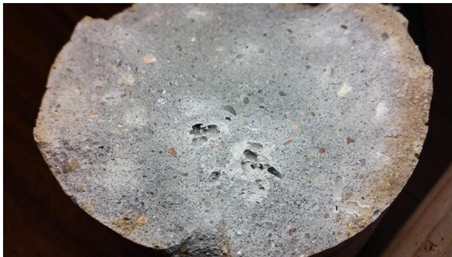
Figure 7. Undissolved chemicals in the mortar
